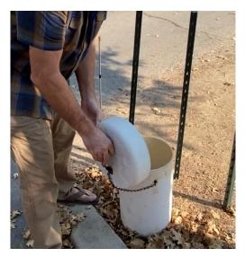
2. Now you can turn ON the water valve in the large, white PVC cylinder by the road at the front of the driveway. Use your legs to keep the cylinder in place while pulling the top off as it can come up from ground. Note: Sometimes it will be buried under snow, and the cap will be frozen. Just heat some water in microwave and pour on cap.
