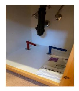
1. Go to Master Bath. Look under LEFT Sink and CONFIRM that the RED/BLUE valve handles are in the 3:30 position. If you don't do this step, the water will be gushing out of the drain line on the side of the house!
